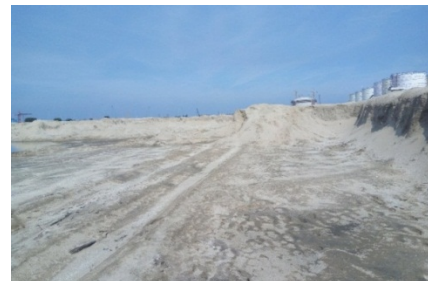
Fig.1 Dredged sea sand at Ennore Port
