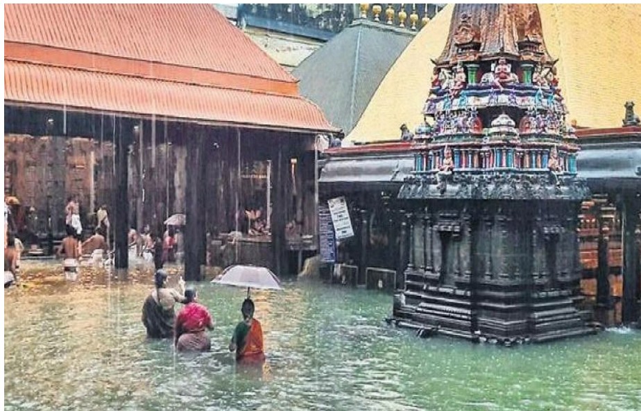
Fig. 2 Temple at Chennai after the cyclone effect
