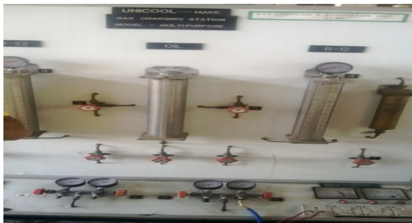
Fig. 9 Installation of Refrigerant in Compressor
