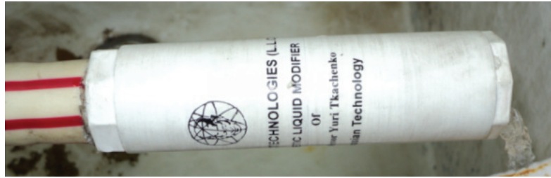
Fig. 6 Installation of MWC-04
